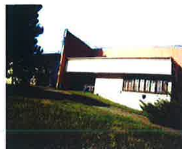
Station de pompage
